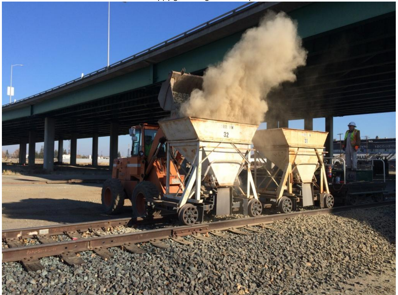
Alan in the loader filling a ballast hopper
