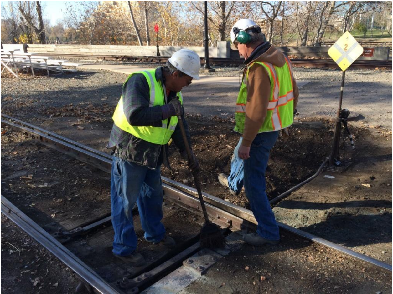
John and Steve work on Switch 2
