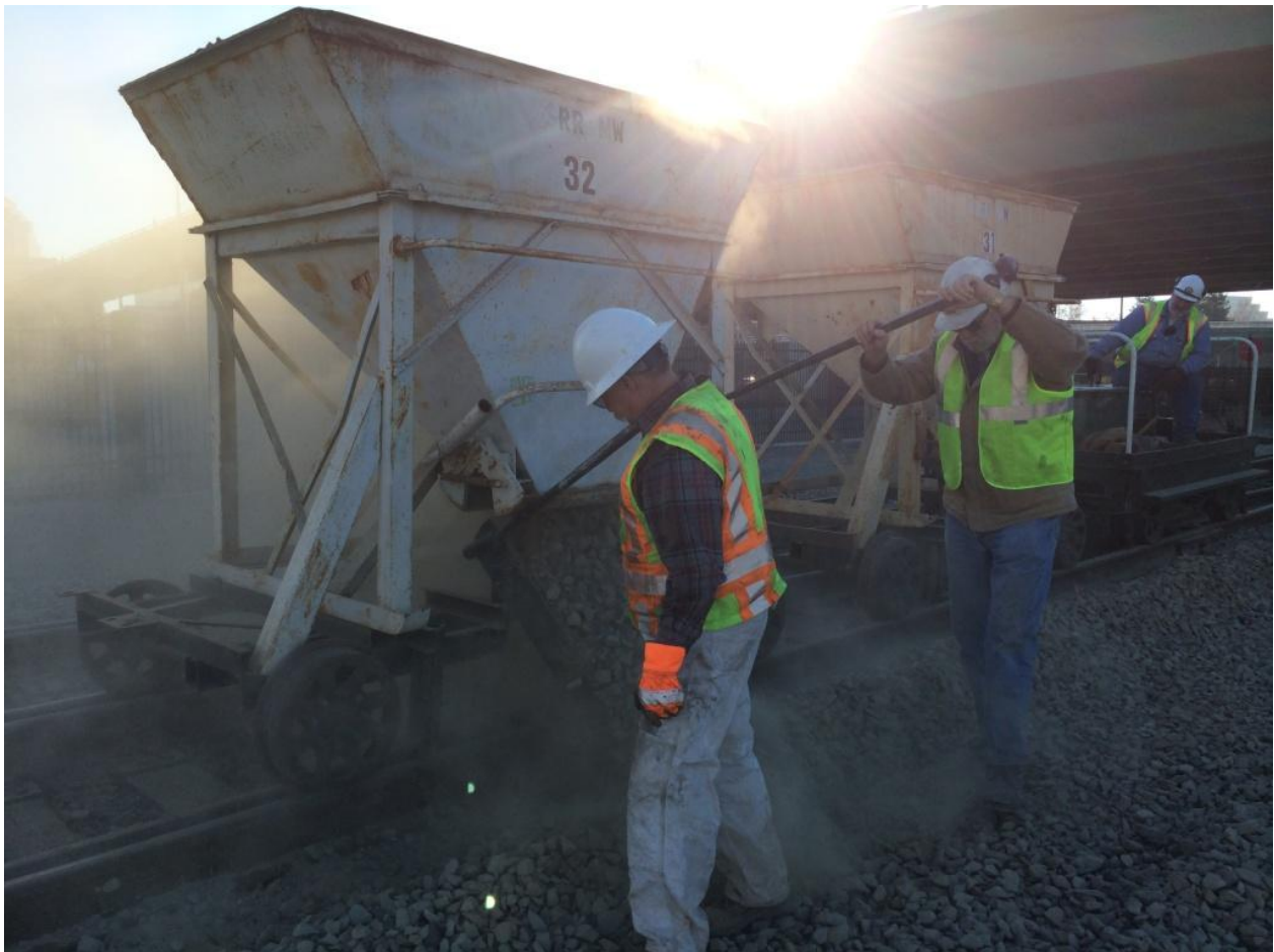
Mike H. and Alan control the flow of rock from the hopper while Frank controls the speed of the operation from the A-6
