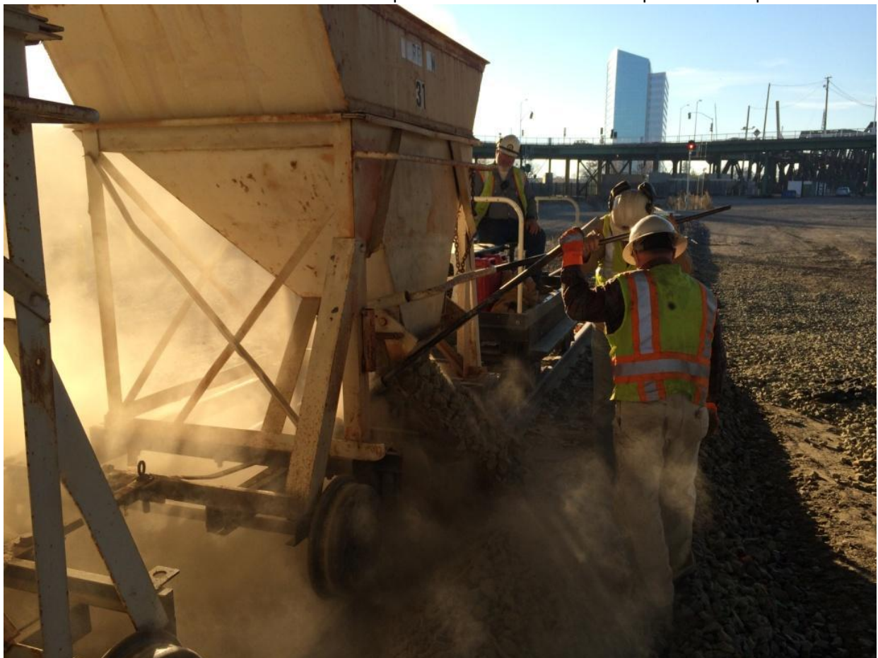
The base layer is laid
